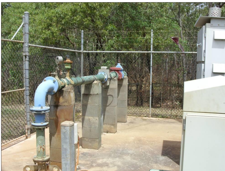
Picture of GA1 showing the raised bore head, concrete slab and fencing.
