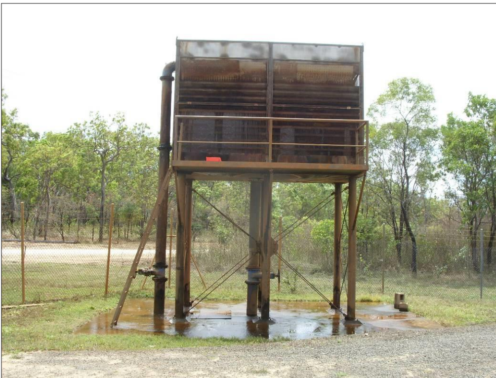
Picture showing the aerator used for iron control.
