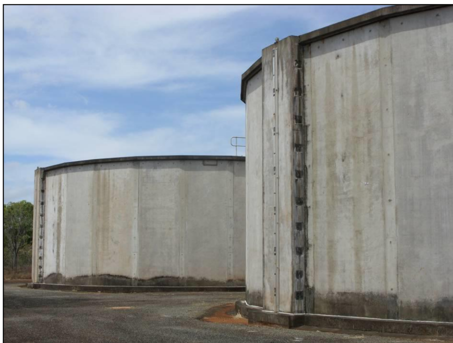
Picture showing the two reservoirs.
